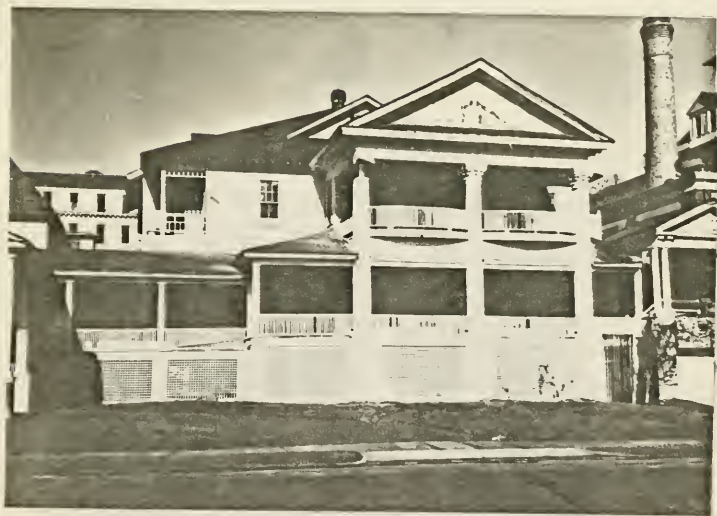
Plate 35: Cottage #3, South Elevation, 1985
